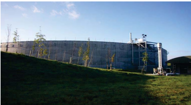
Dairygold's anaerobic digestion plant at Castlefarm, Mitchelstown, Co. Cork
