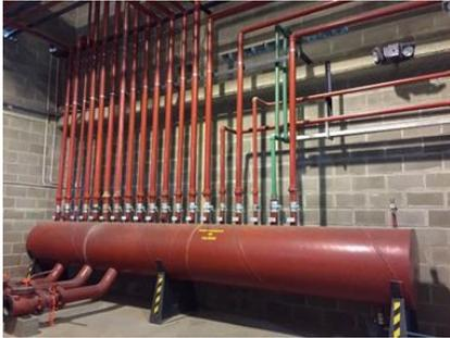
*Boiler piping that distributes hot water for heating in plant 6. Energy source was replaced from packed gas to supplied natural gas*
