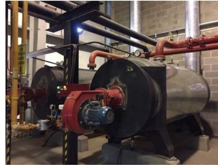
*Boiler burner in plant 6. Energy source was replaced from packed gas to supplied natural gas.*
