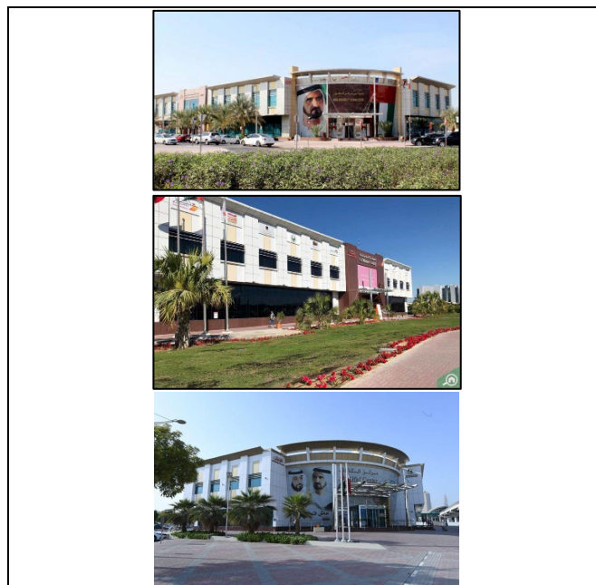
Dubai Municipality – Twar (top), Manara (middle) & Kifaf (bottom) Buildings
